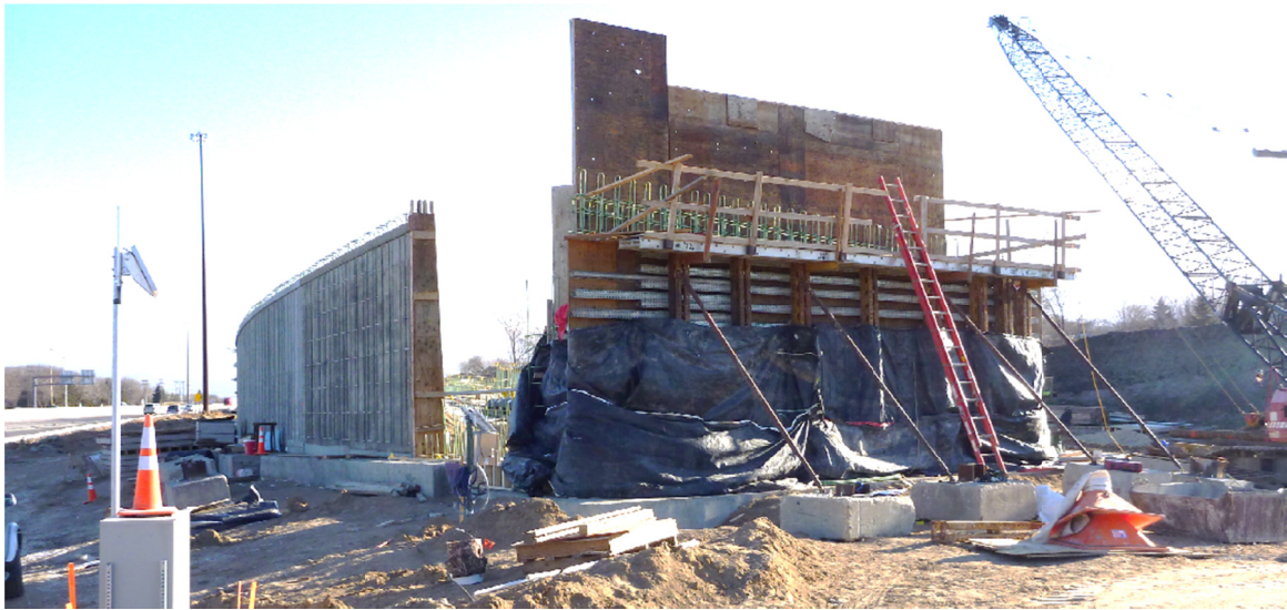
Figure 5. The BR 27V97 north abutment pile cap has been cast; formwork is in place to cast the abutment stem; a portion of the north retaining wall is in place.
