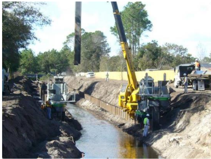
Figure 11. Clamp Crane Pitching Sheet Piles to Press-in Pile Drivers
