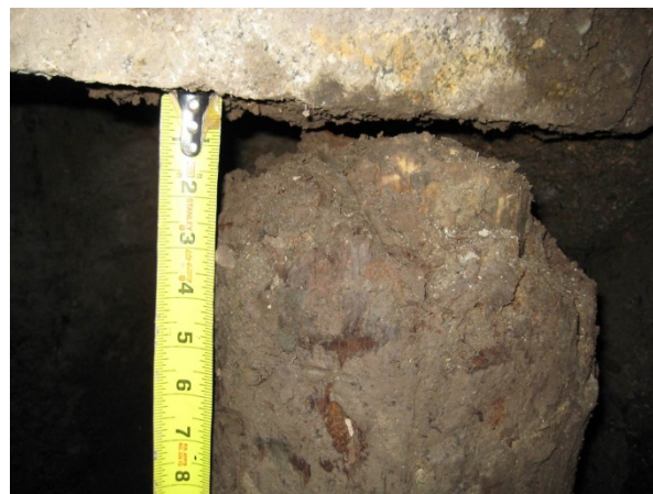
Photo 2: Deteriorated Top of Timber Pile Under the TOMC Bell Tower Foundation Wall.
