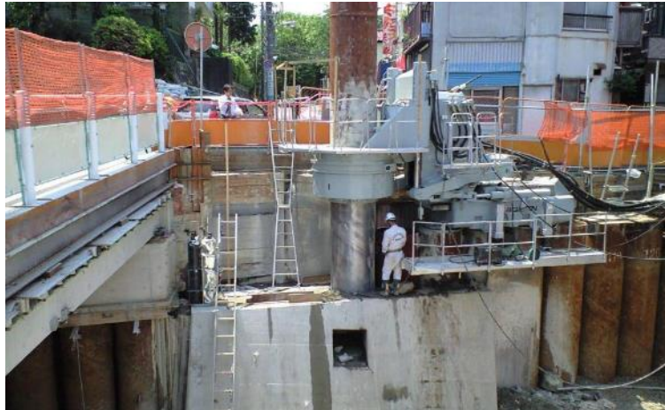
Figure 15. Gyro Press Piling Directly into Concrete Bridge Abutment
