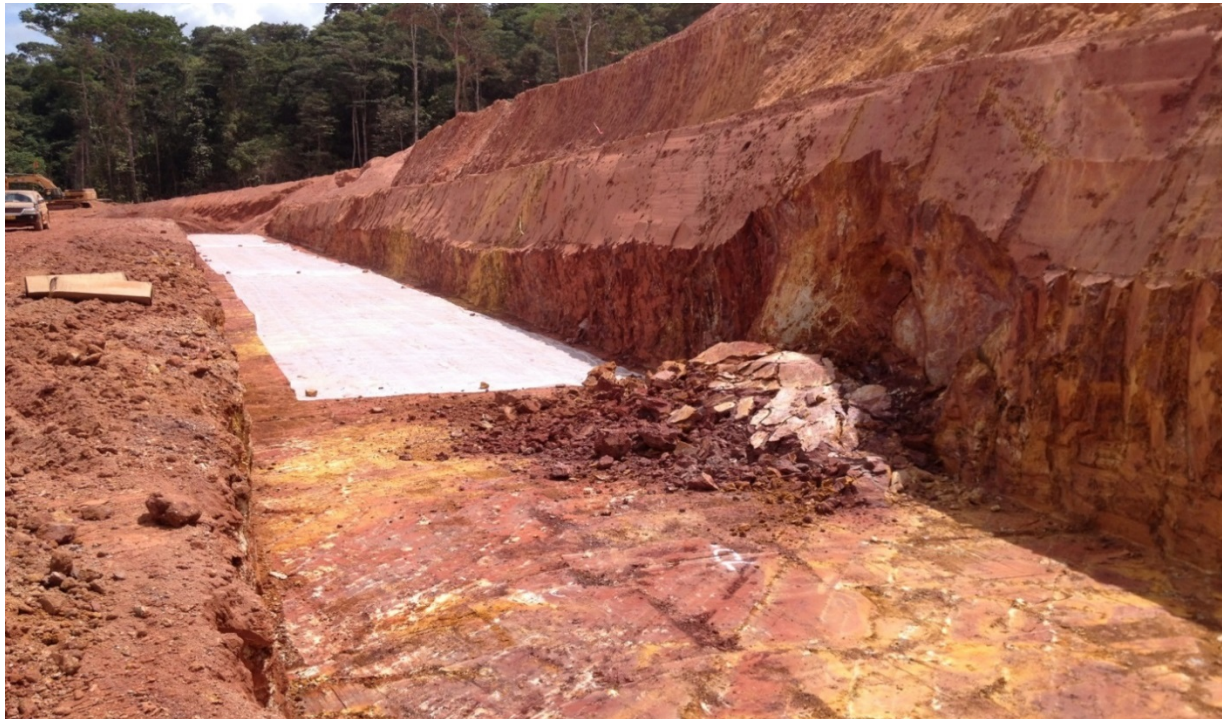
Figure 12. View of site preparations and SAPROLITE side fill.
