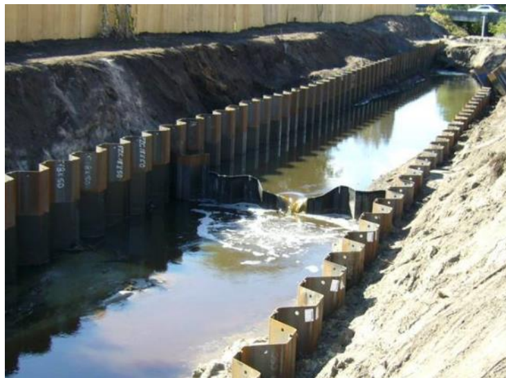
Figure 12. Driven Sheet Piles
