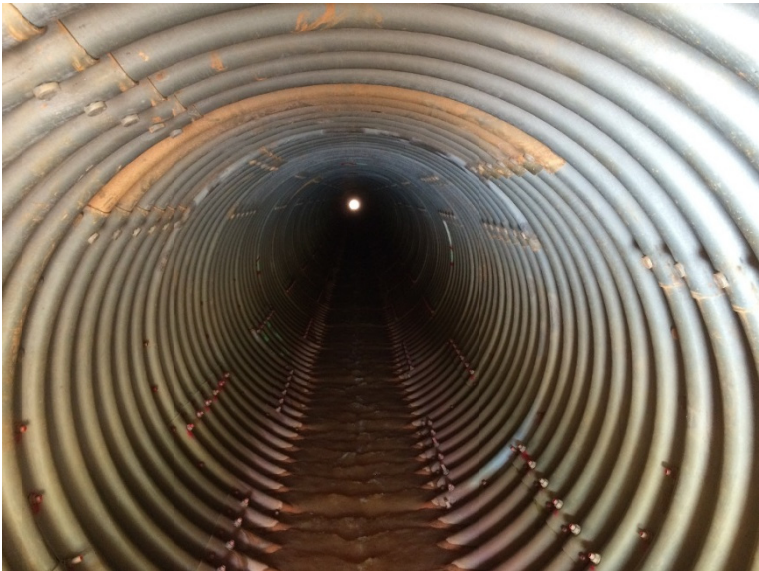
Figure 16. Interior view of the in service culvert.
