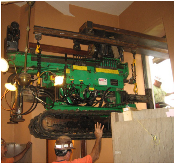
Photo 3: Micropile drill rig hoisted through window into the bathroom.
