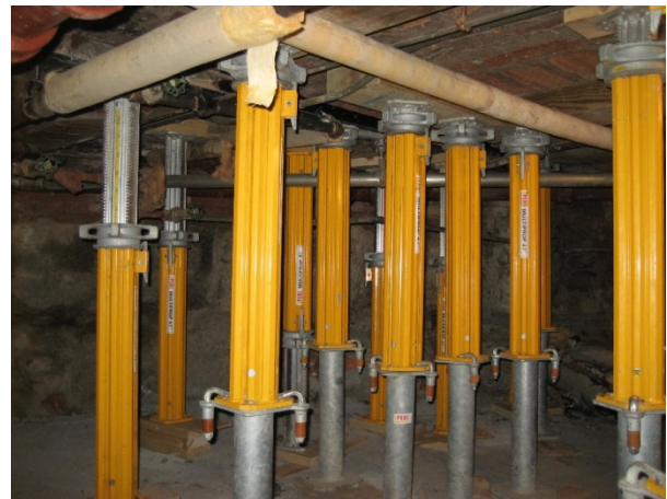
Photo 4: Shoring posts installed below bathroom along path of rig travel.
