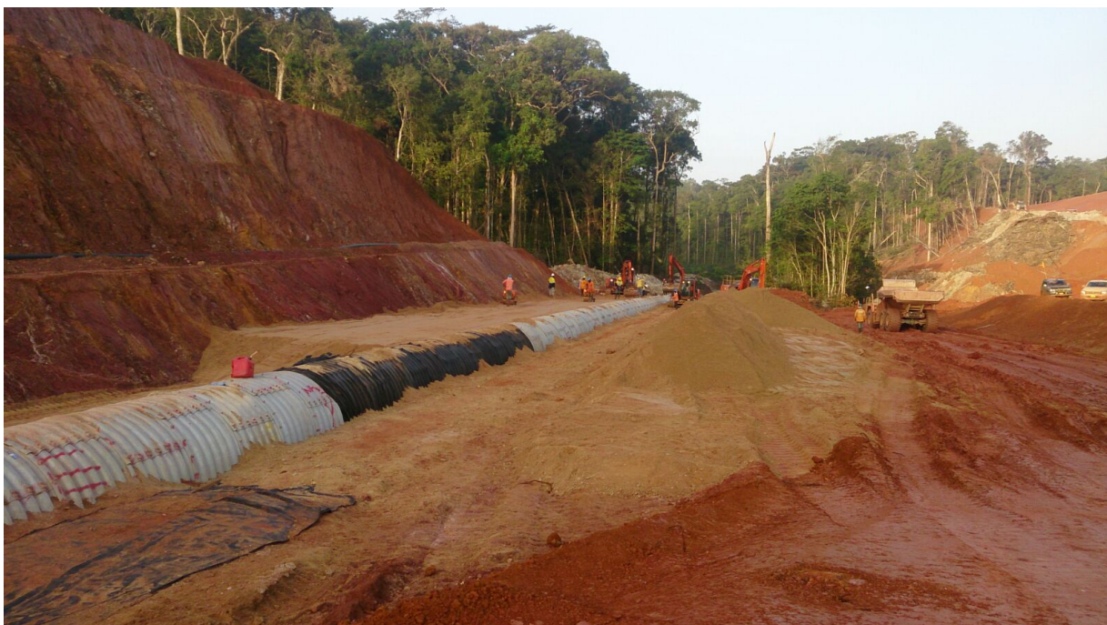
Figure 13. View of culvert, sand backfill and sloped saprolite.
