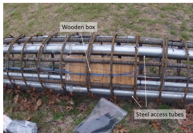
Figure 4. A photograph of the wooden box tied on the rebar cage
