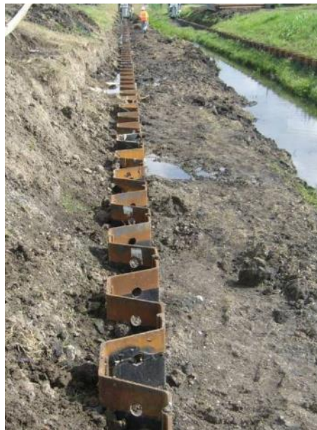
Figure 8. Alignment of Pressed-in Sheet Piles
